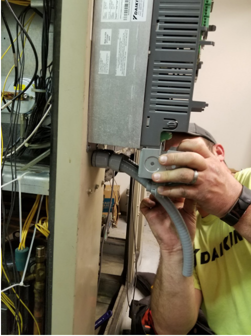
Figure 5: Actuators for Waterside Economizer
